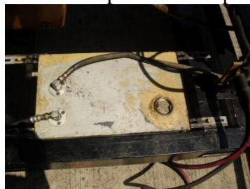
Gambar 3. Fuel tank tanpa vent
